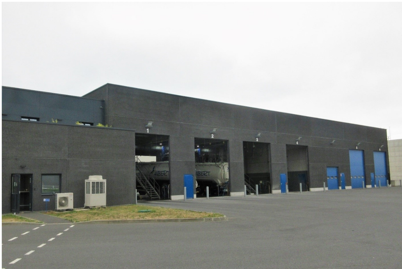
Station de lavage
